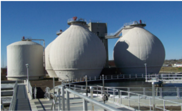
Anaerobic digesters at the Lincoln, Nebraska wastewater-treatment facility
