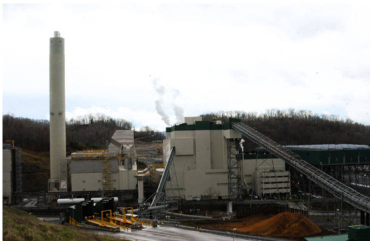
Exterior view of the Virginia City Hybrid Energy Center (610 MW) in the Town of St. Paul, in Wise County, Virginia.
